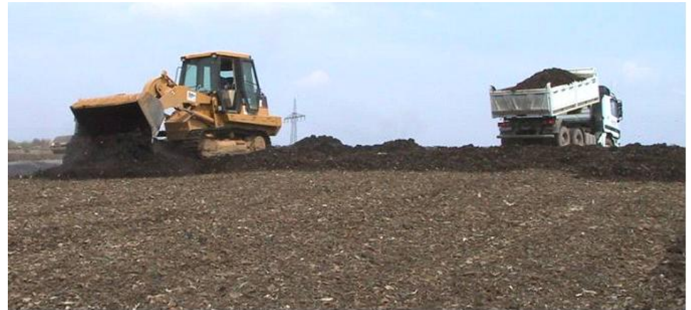
Placement of Methane oxidation material
