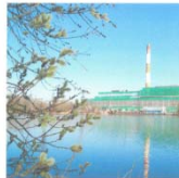
Thermal power plant, Russia
